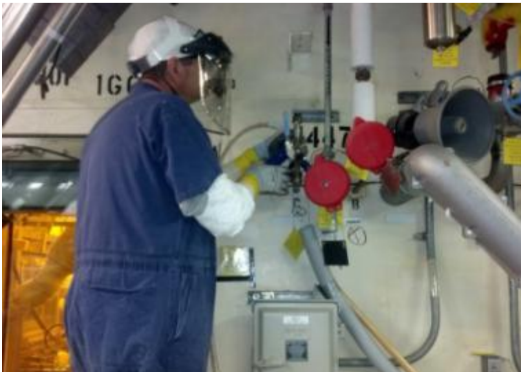
Vitrification Cell Wall Penetrations Stabilization
