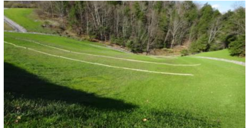
Lake 2 After Completion of Dam Repairs
