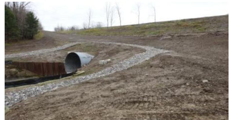
Final Grading of the Buttermilk Creek 18-Foot Culvert Slope
